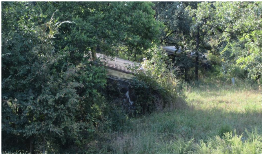
Figure 4.5-A view of old Fountainhead cabins on HW 150
